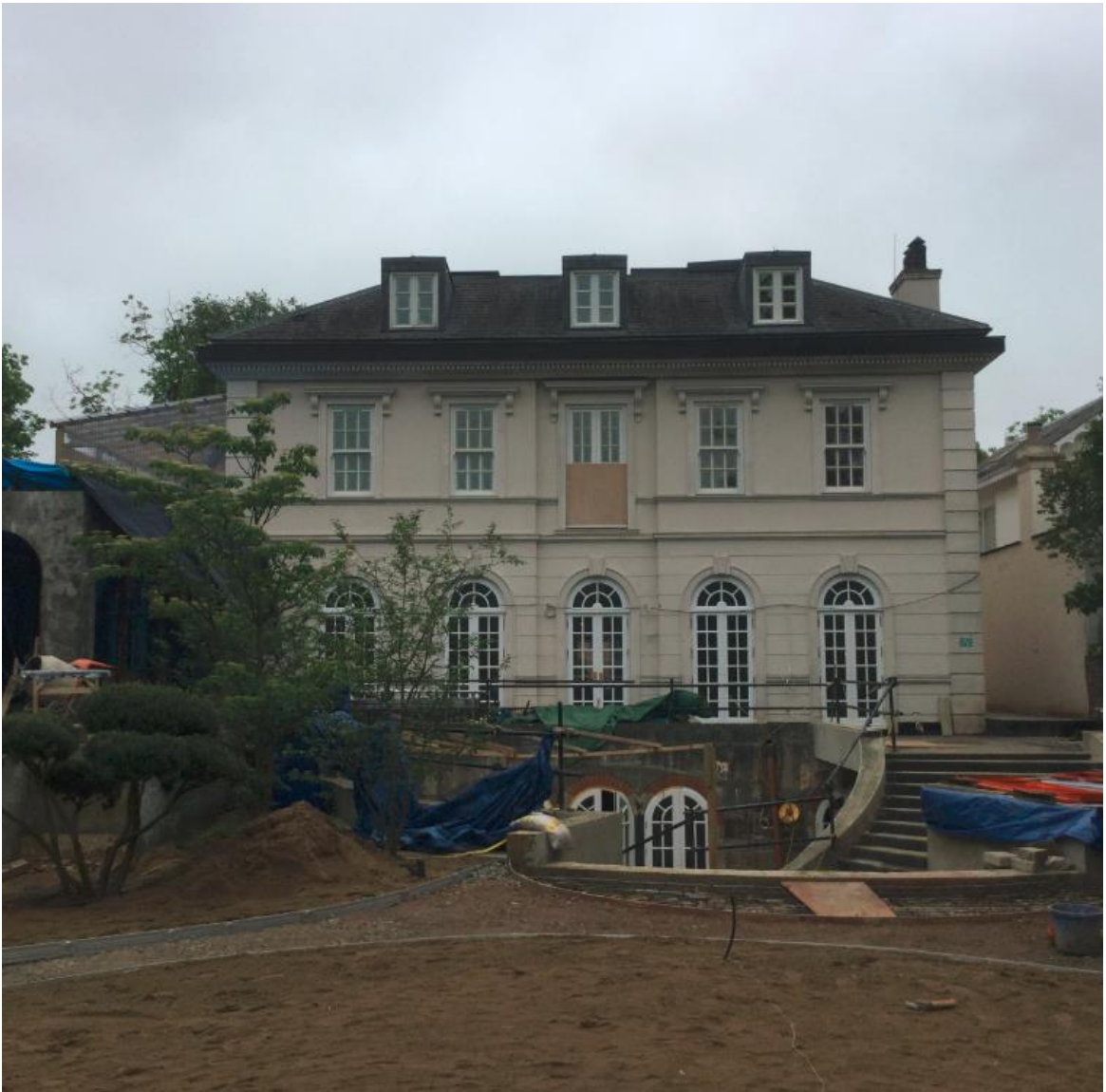
Rear of subject building.
